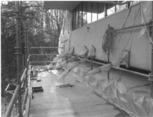
Figure 68: Preparing the cables in the beam for prestressing
