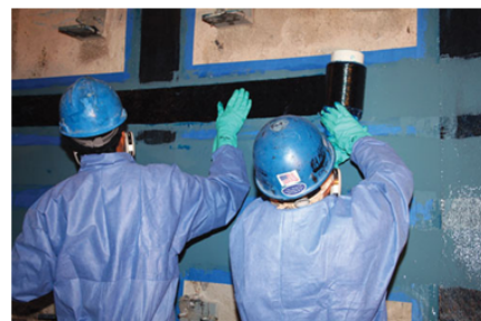
Figure 60: Carbon-fiber reinforcement of the walls of the sixth-floor ramp.
