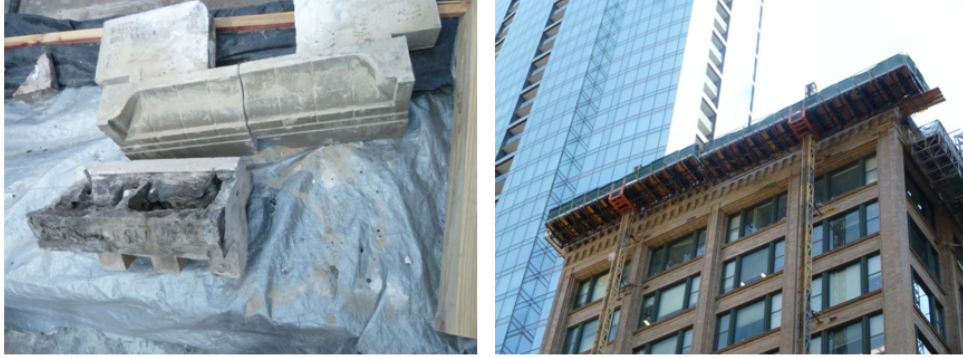
Figure 87: Detain of a terracotta cornice on the renovation worksite at the University of Chicago. Mary Brush, Preservation Architect, Holabird & Root
