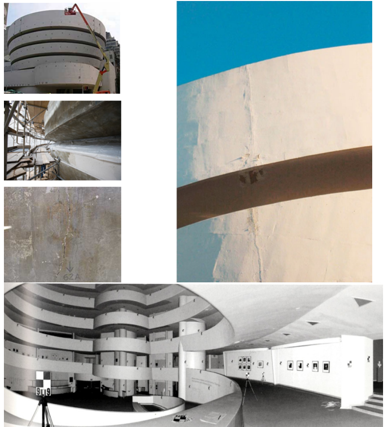
Figure 58: Structural analysis to determine the way the building had shifted
