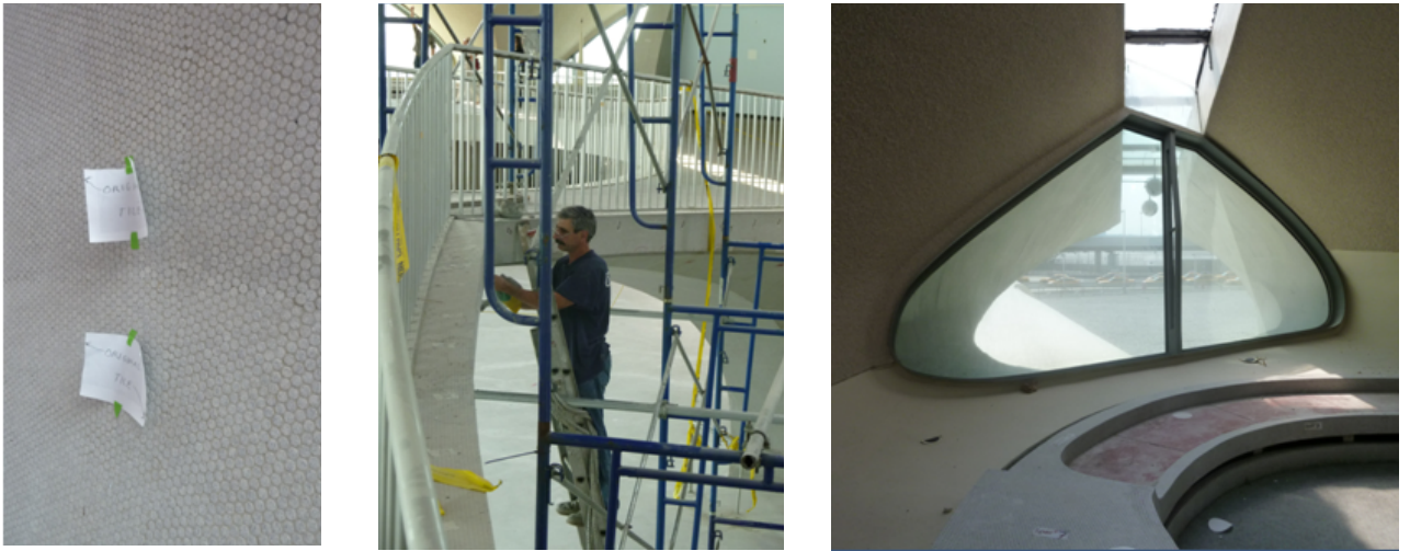
Figure 88: Renovation of the TWA Terminal at JFK Airport, New York. The ceramic tiles had to be carefully replicated for the repair work, with meticulous execution by workers similar to that for a precious mosaic. Renovation of the he highly complex curtain walls was made possible by custom recreation of the neoprene joints (gaskets)
