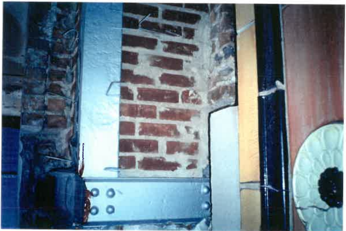
Detail of the wall structure showing the glazed terra cotta veneer hooked to the metal structure and the brick bearing wall.
