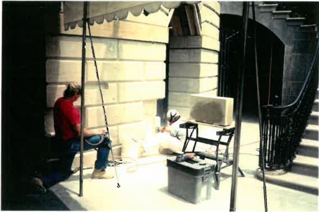
Restoration of the facade by the stonecutters (use of mechanical tools)
