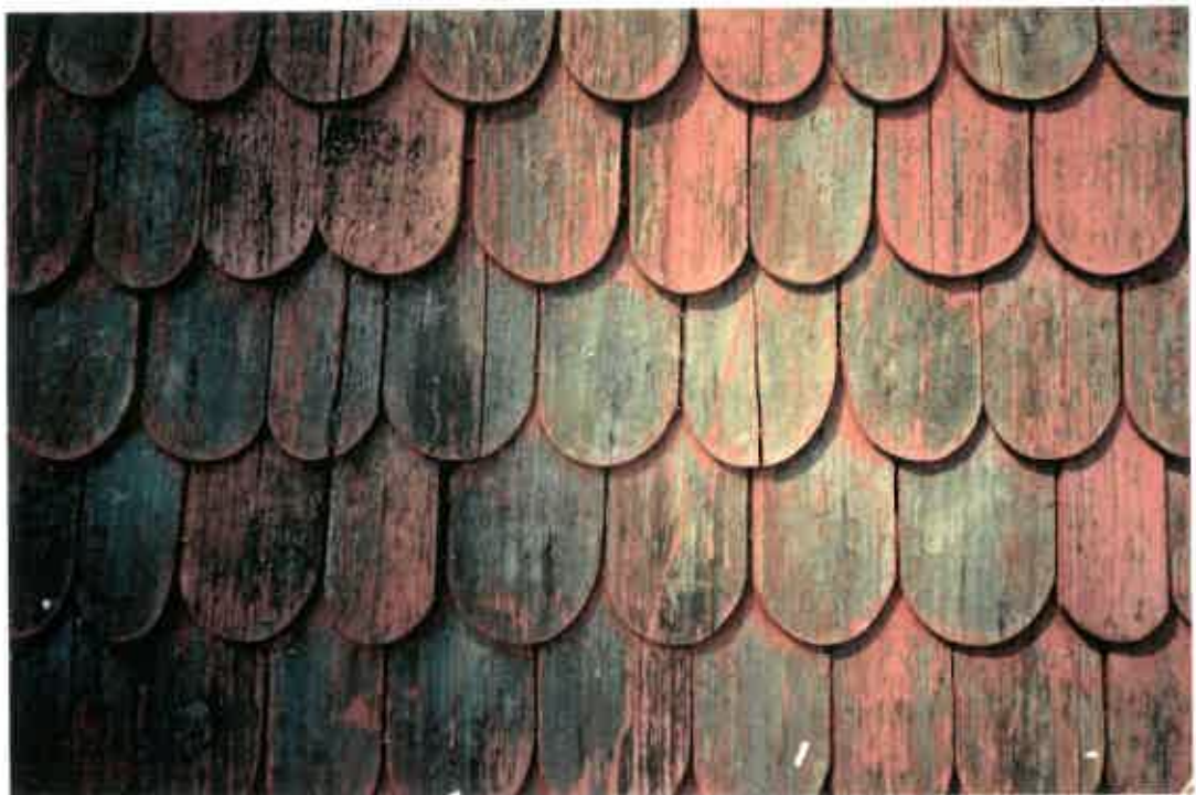
Shingle roof of the mansion house, using red cedar elements as a substitute material to the original bald cypress one, no more available. Painted in "spanish brown" colour.
