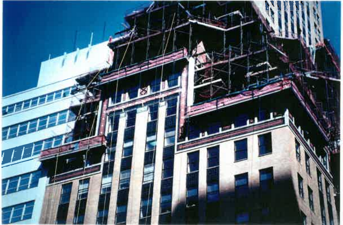
Glazed terra cotta elements decorating the facade along the edges and the window sills.
