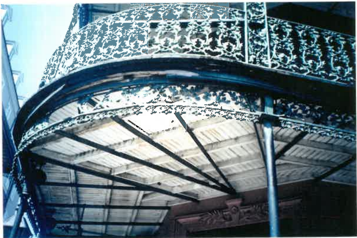
View of the gallery , using cast iron ornated elements, and wrought iron radiating bars to sustain the wood beams and deck.
