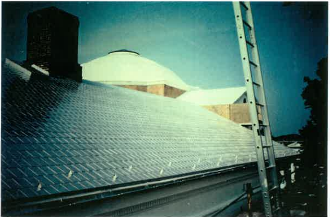
Newly restored pavillon with its tinplate roof recovering the original metal roof kept underneath.
