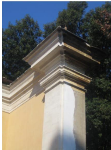
Villa de Medicis, Roma, Italy. restoration architect: Didier Repellin, ACMH
