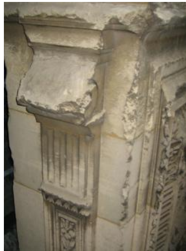
Court Visconti, Palais du Louvre, Paris. Restoration Architect: Michel Goutal, ACMH
