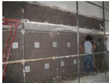
Mortar Injection Process, Villa de Medicis, Rome. Didier Repellin, ACMH
