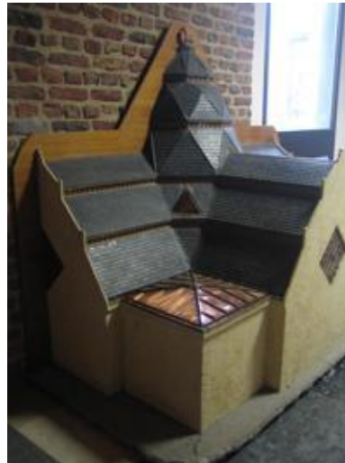
The master work of a Compagnon in Lille. the scale model is a slate and copper roof.
