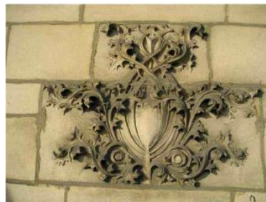
The Gage Building, Chicago Illinois. Architect: Holabird and Roche with Louis Sullivan. Restoration Architect: Mary Brush, Klein and Hoffman
