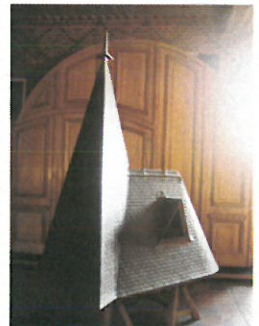
Compagnon Maquette: ardoise (slate) roofing
